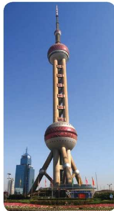
▲ The Oriental Pearl Tower in Shanghai is over half a kilometre high. In high winds, its top can move by a quarter of a metre. But, being elastic, its steel and concrete structure always returns to its original shape.
